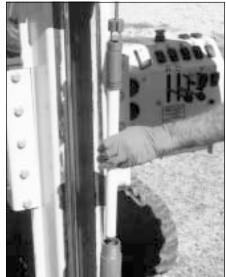
Figure 3. Screen assembly is lowered into position with extension rods.
